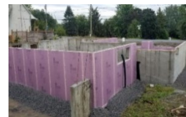
*Exterior basement insulation and drainage system
